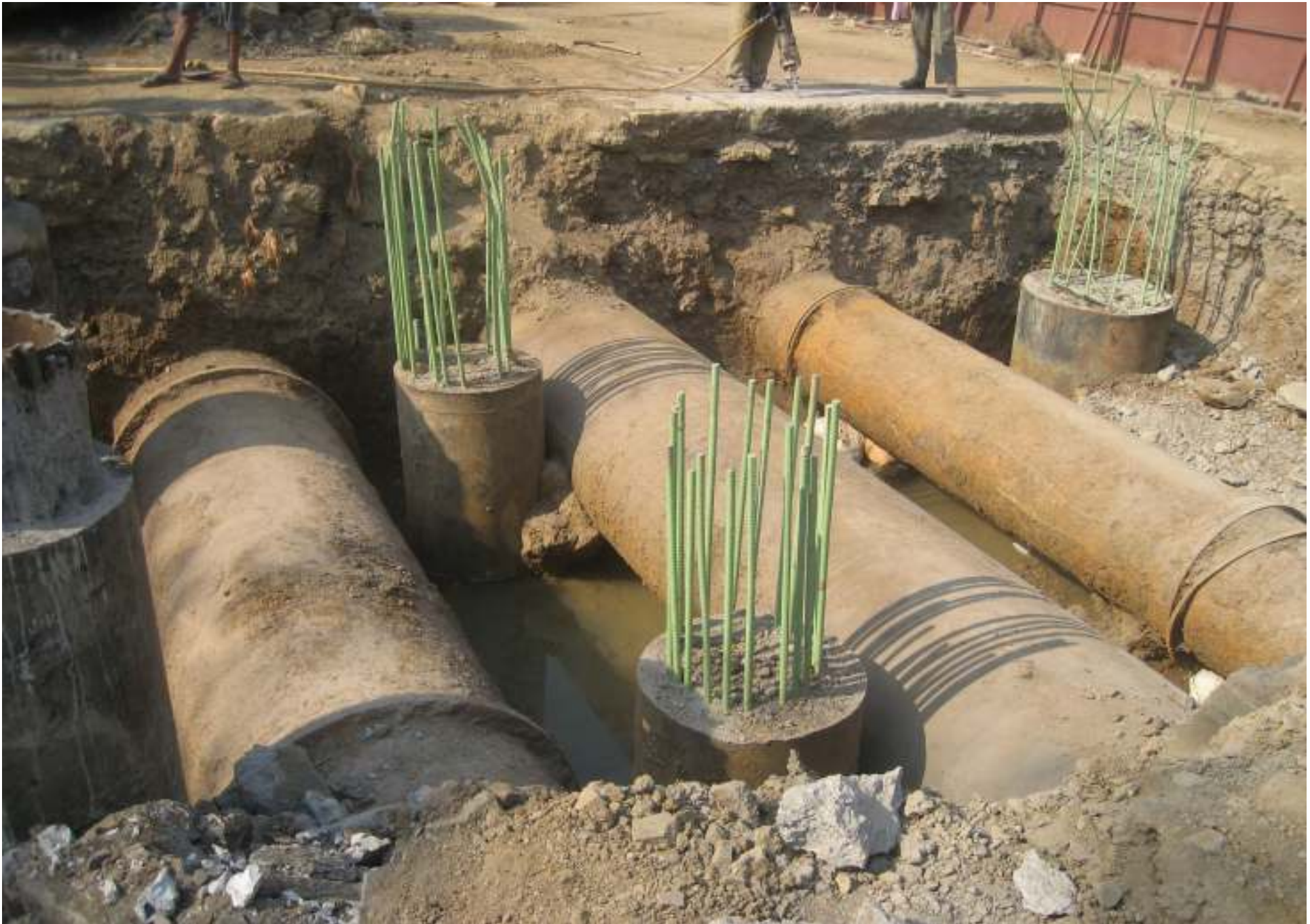
PILING IN DIFFICULT CONDITIONS CREATED BY OLD WATER MAINS
