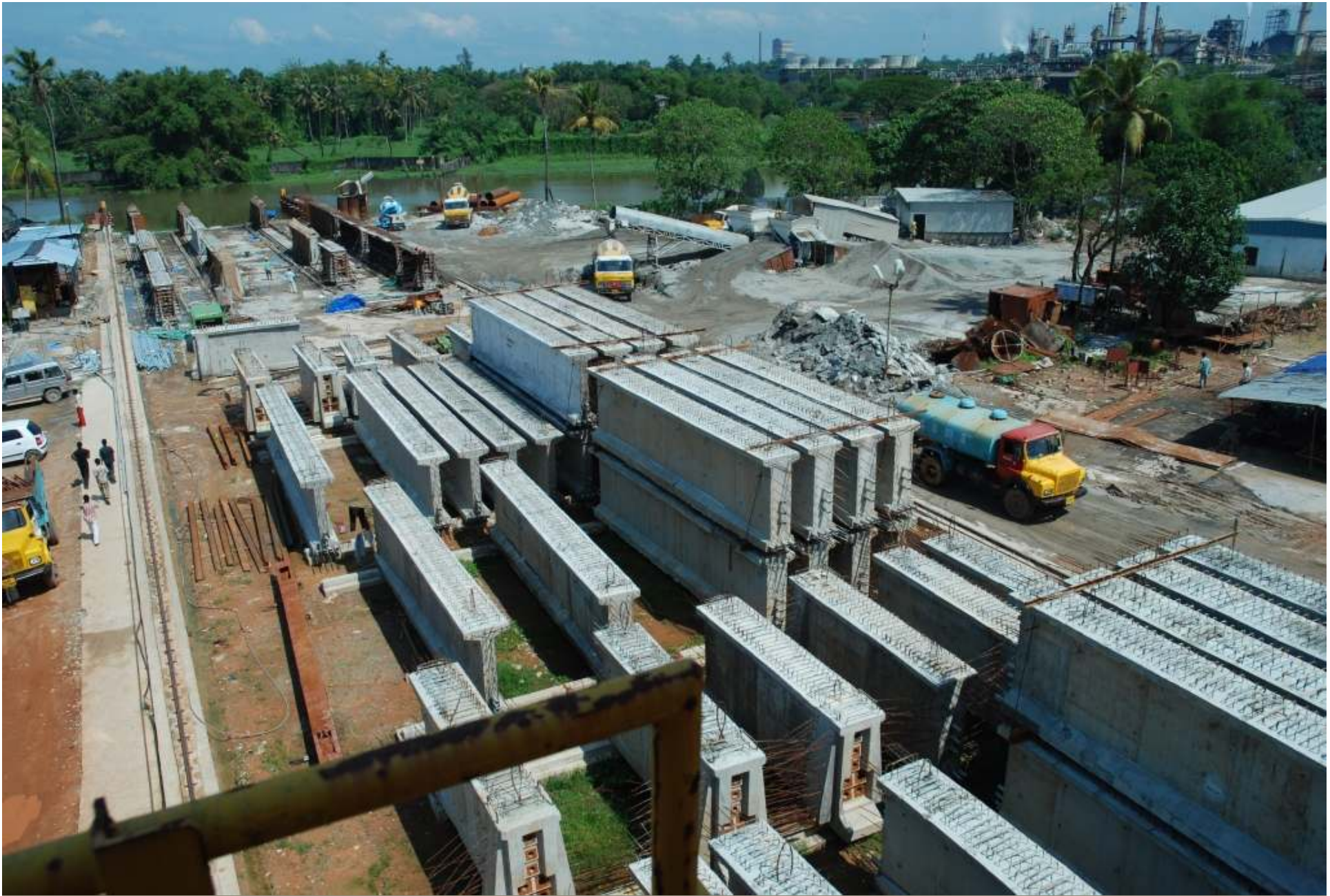
VIEW OF CASTING YARD SHOWING STORAGE OF GIRDER SEGMENTS
