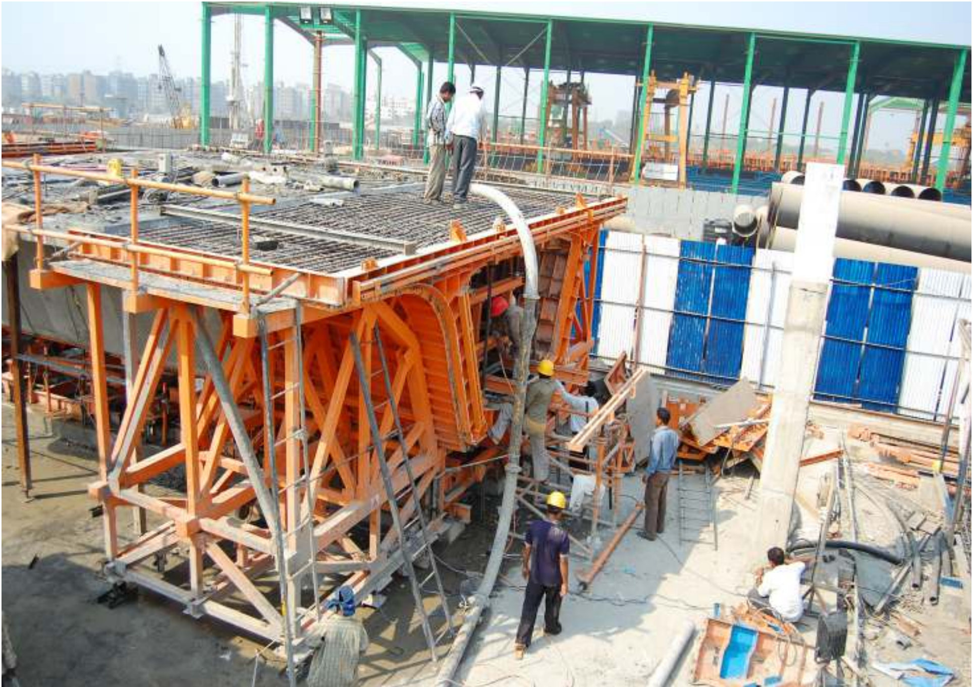
MATCH-CASTING IN PROGRESS
