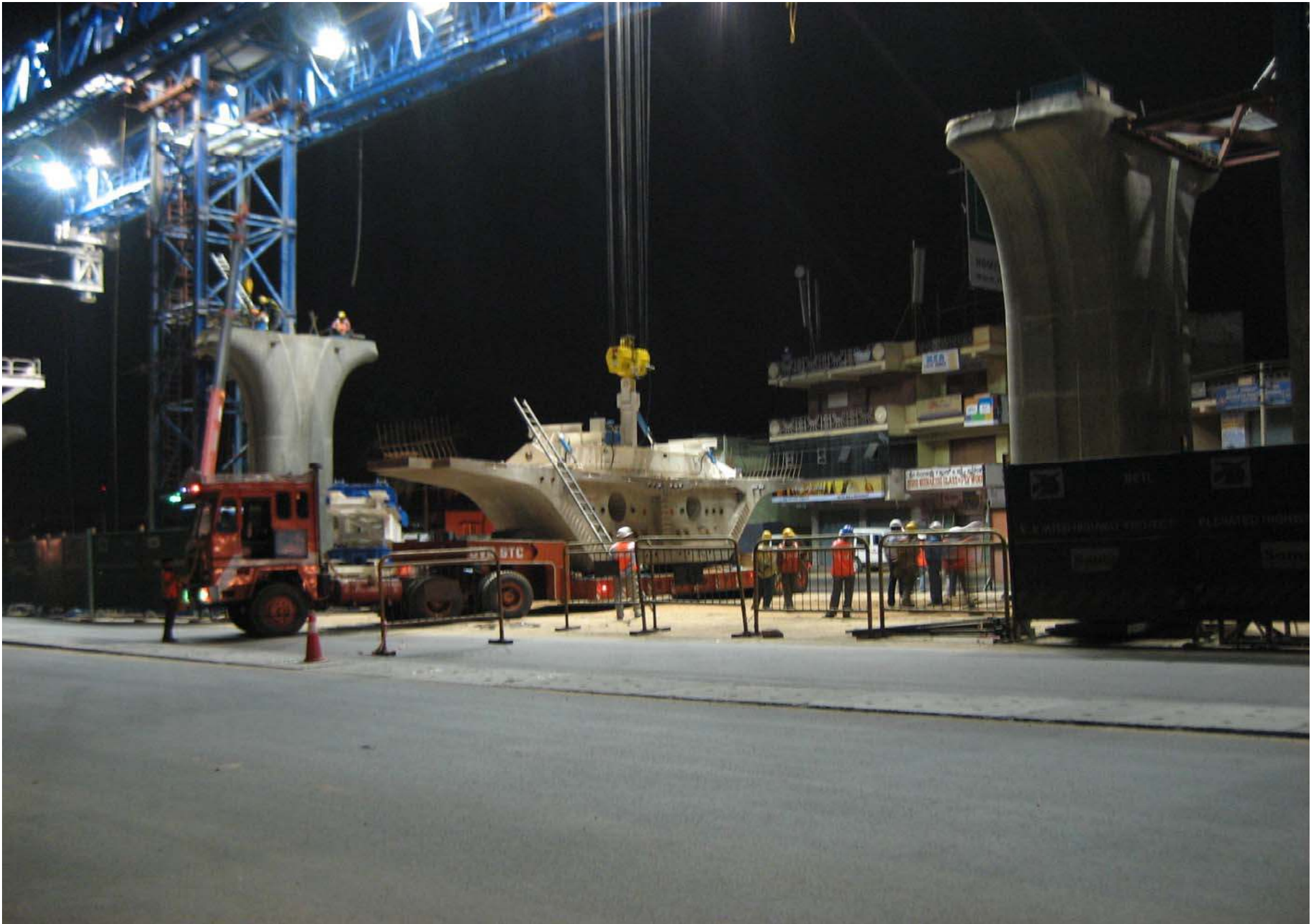
BANGALORE ELECTRONIC CITY X'WAY: SEGMENT ARRIVAL AT SITE
