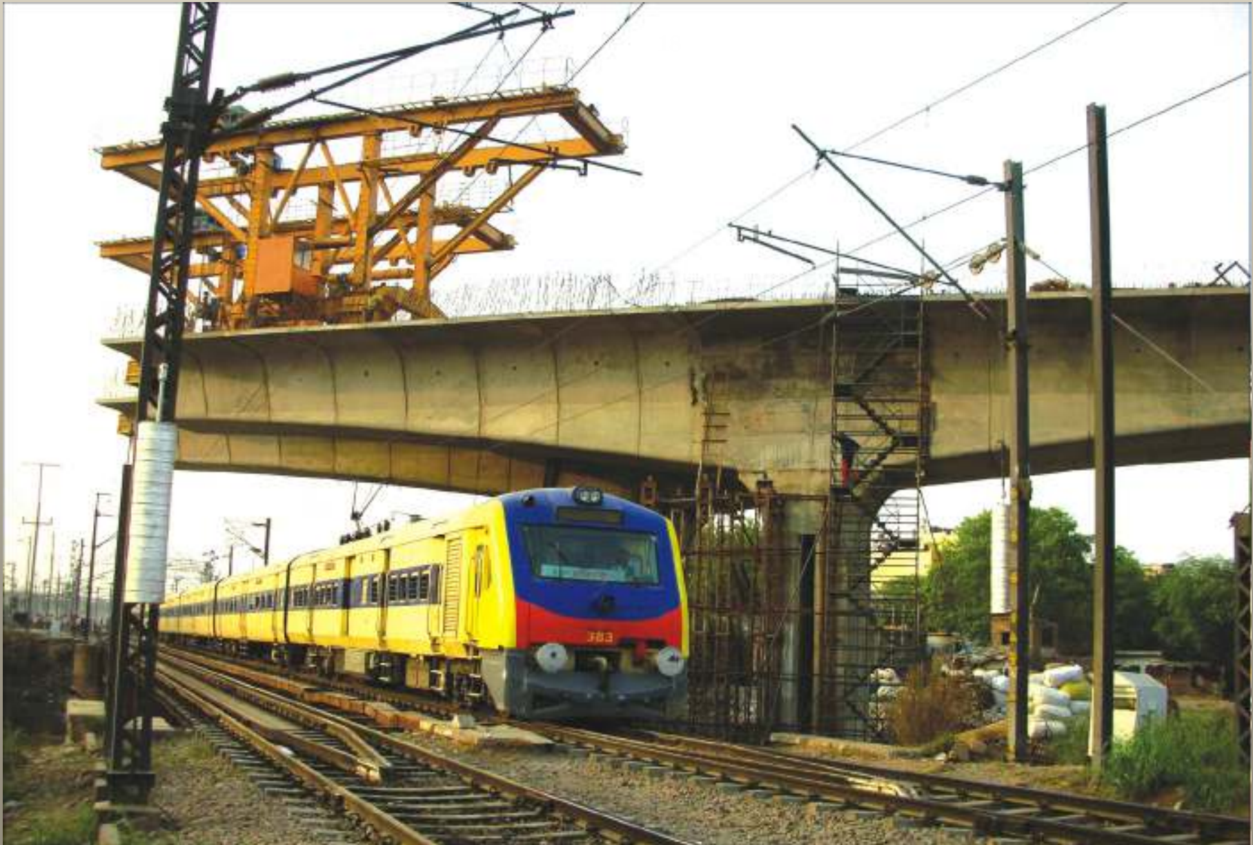
THE RAILWAY CROSSING UNDER CONSTRUCTION OPERATION MIDNIGHT: 2 hrs, alternate days
