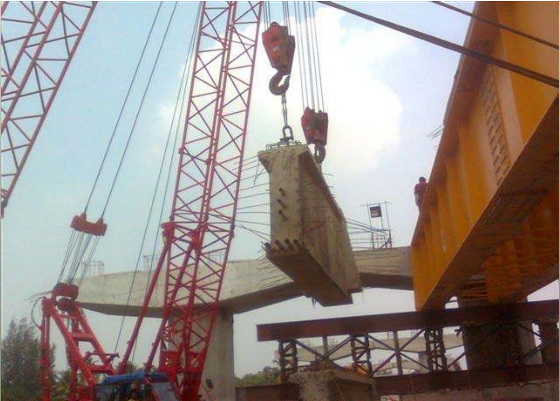
80t BARGE MOUNTED CRANE ERECTING THE GIRDER SEGMENTS
