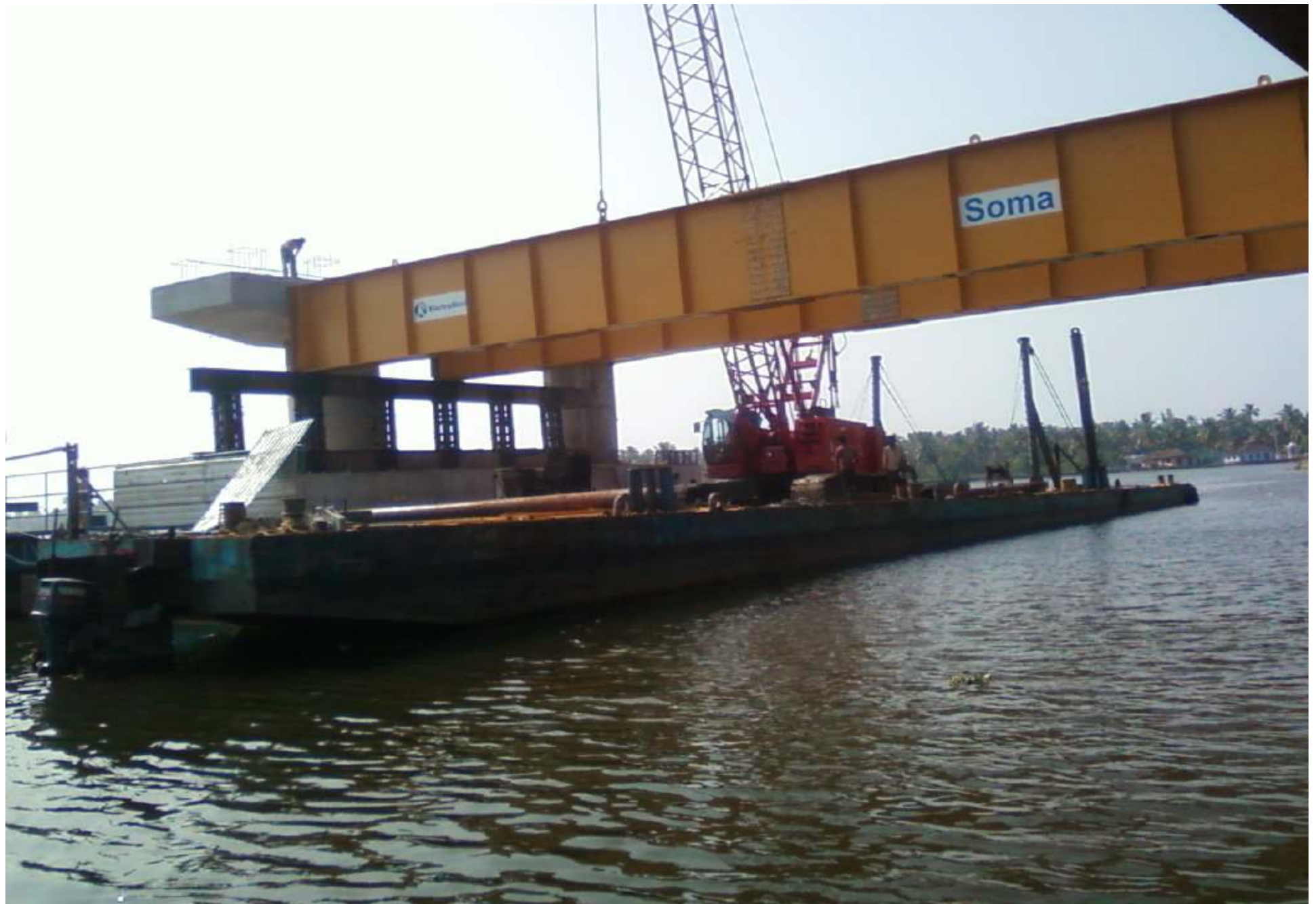
85 t PLATE GIRDERS USED FOR SEGMENT ASSEMBLY
