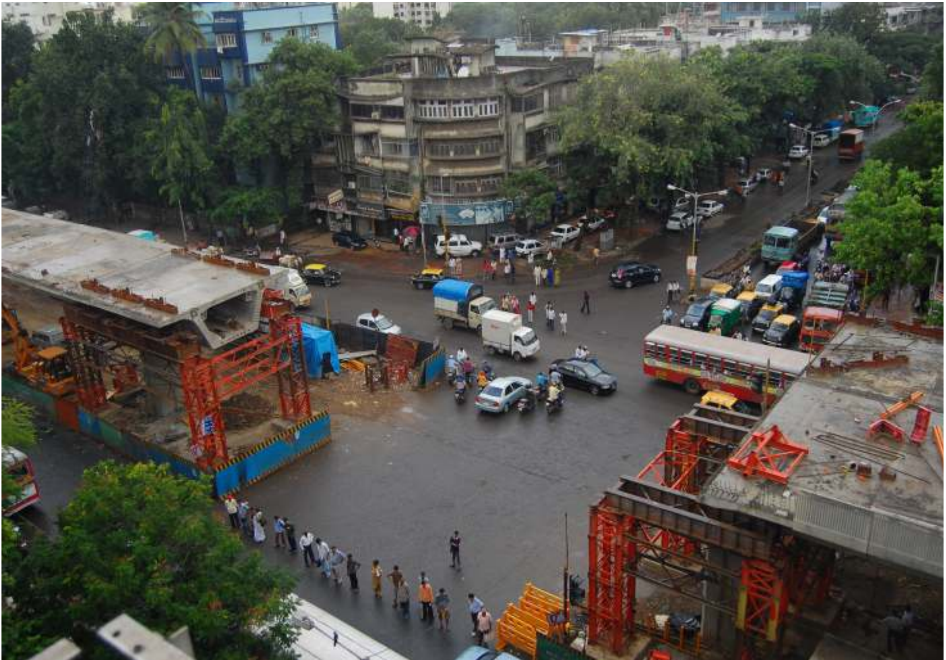
PREPARATION FOR LAST SPAN ERECTION
