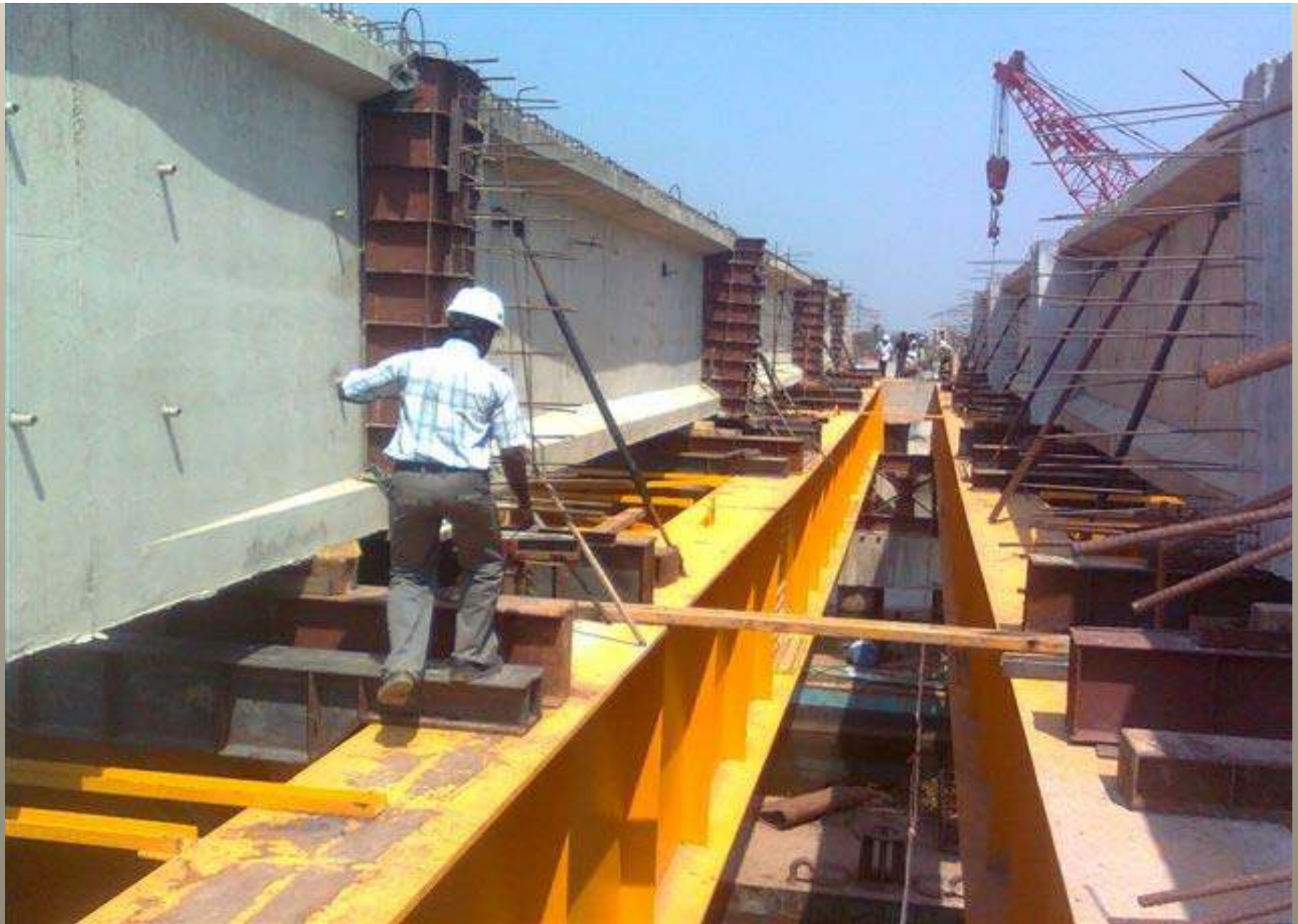
SEGMENT SPLICING AND DIAPHRAGM STUBS
