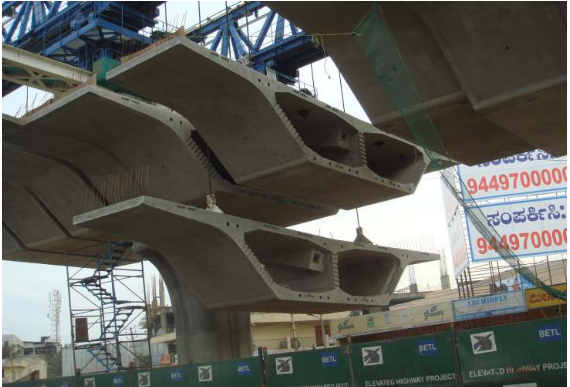
PRECAST SEGMENTS SUSPENDED FROM MAIN TRUSS DURING ERECTION
