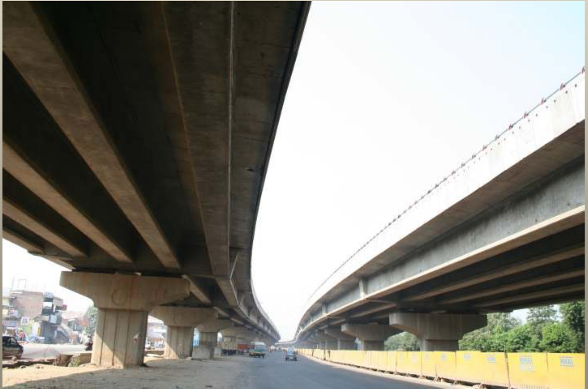
HANGING GIRDERS OF GURGAON: NEARING COMPLETION
