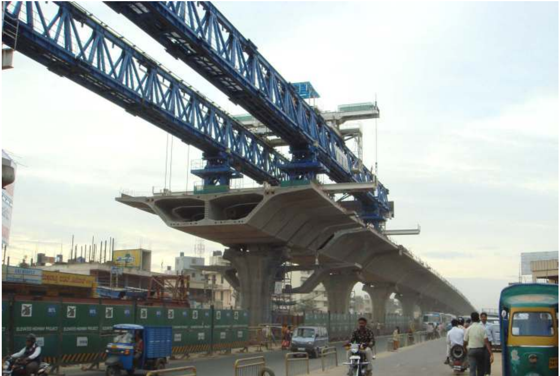
GENERAL VIEW OF PRECAST SEGMENTAL CONSTRUCTION WITH OVERHEAD LAUNCHING TRUSS
