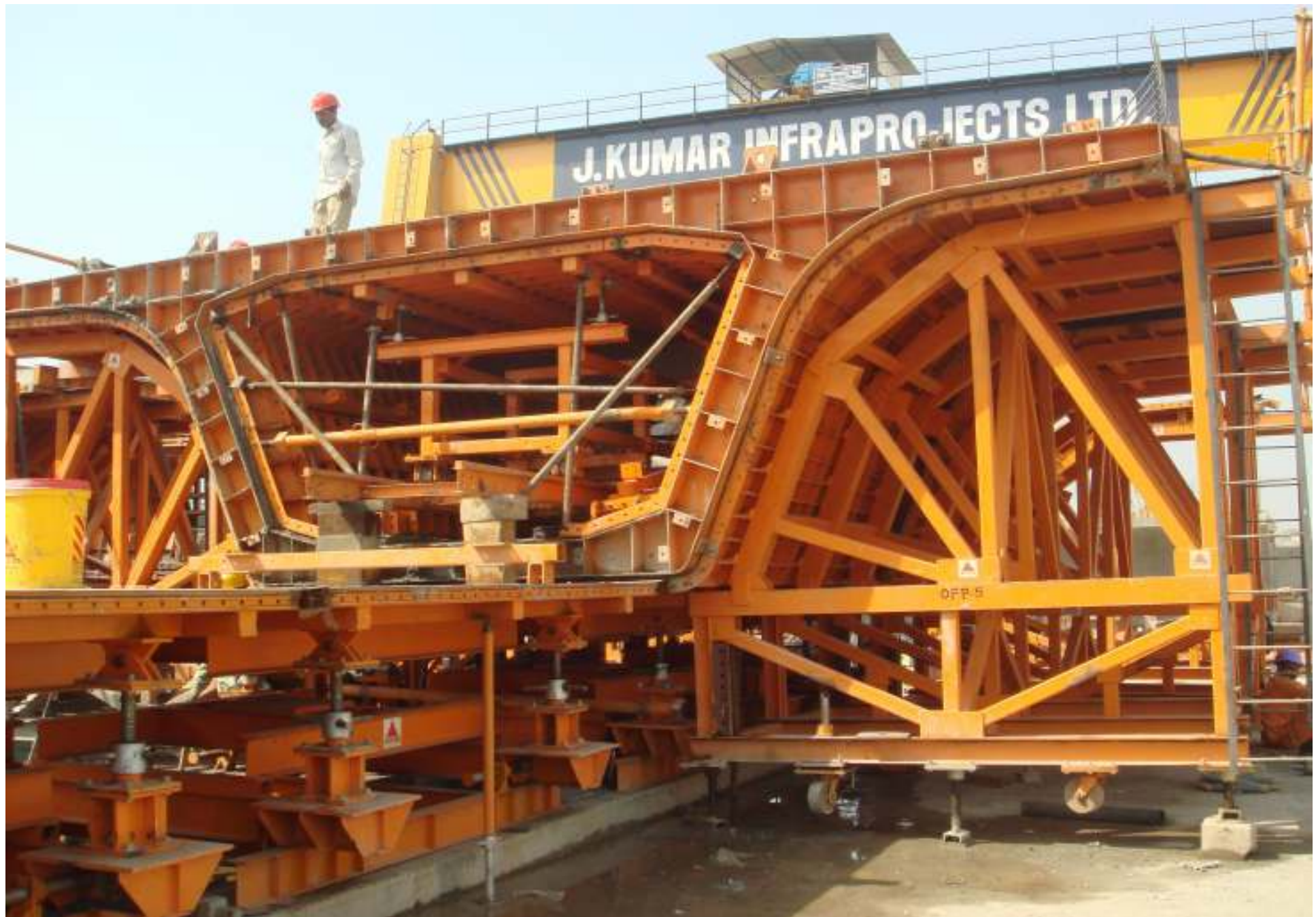
CASTING YARD MOULDS WITH ADJUSTABLE BED
