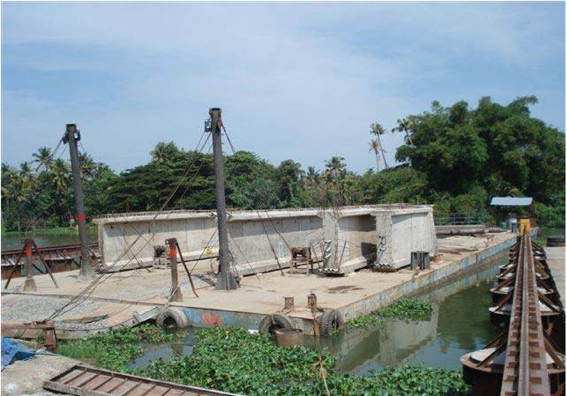
GIRDER SEGMENTS Wt 30t EACH
