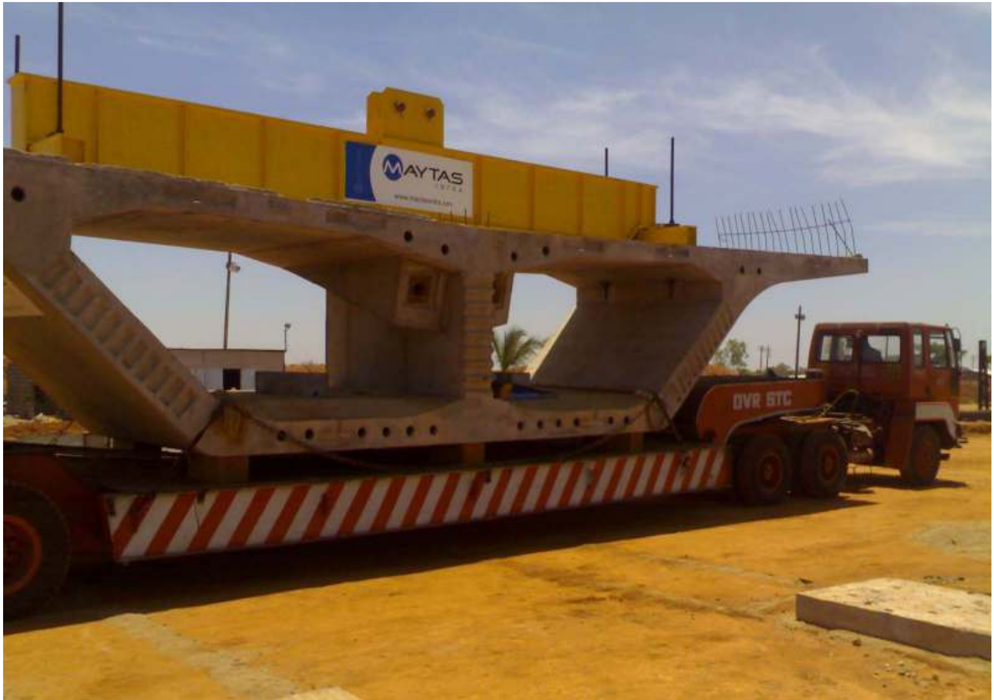
PRECAST SEGMENT TRANSPORTED BY LOW BEDDED TRAILOR TO SITE
