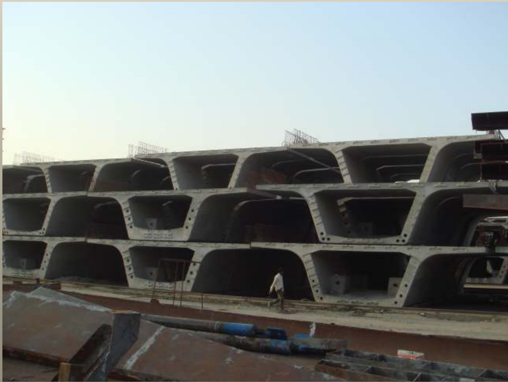
CASTING-STACKING YARD
